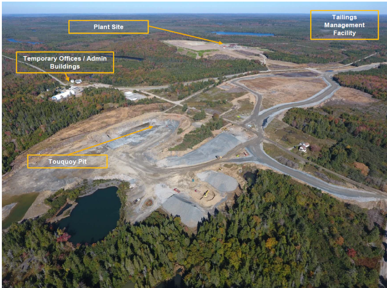
Touquoy Mine site; aerial
