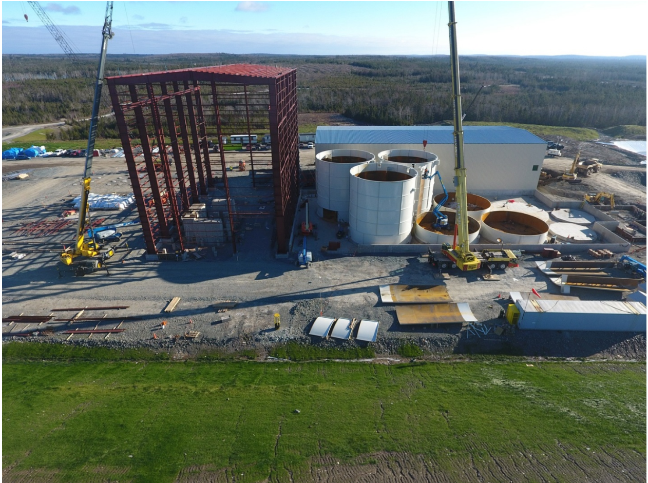
Touquoy project; Steel structure for grinding building
